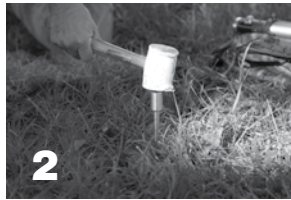
2 Drive in spike with rubber mallet.
