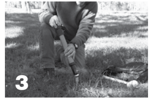
3 Thread the coil base into the spike.
